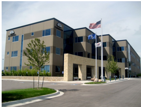
Recently completed Building 4 at 119 th Street and Renner Boulevard in Olathe.
